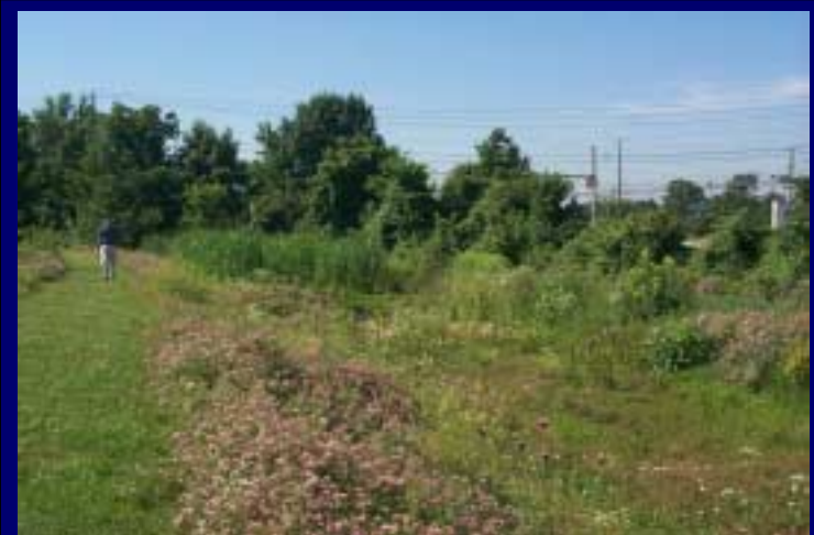
Pollutant laden stormwater is conveyed to this beautiful and functional constructed wetlands, to benefit from phyto-remediation and infiltration.
