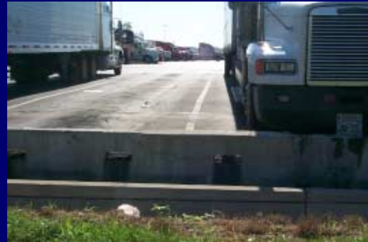
Runoff from parking lot is collected through a trough system that settles out black tire dust and debris
