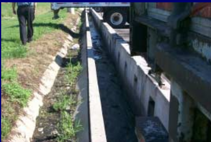
The trough system conveys stormwater to a wetland treatment system
